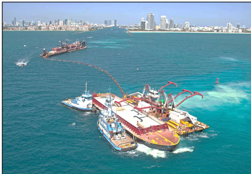
Figure 10. Aerial view of the Cutterhead Dredge Texas working in the offshore channel during the PMDP. Spider-barge loading dredge material into transport scow for disposal shown in the foreground. Note the plume of turbid water discharge from the overflow valves on the scow. Dredge plume is being carried north by prevailing surface currents. At the top of the photo is the cutterhead dredge swinging across the channel. Note the much smaller turbidity plume created by the cutterhead that is confined within the channel boundaries. Plume movement within the channel is dominated by east-west tidal currents. View is looking west. Photo courtesy of Great Lakes Dredge and Dock.
