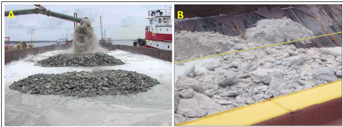
Figure 9. Photos of dredge material being loaded into scows. (a) During CSD operations with suction engaged, the dredge slurry contains a mixture of water (90%) and cut rock (10%). The rock fragments are all < 33 cm in their longest dimension. Note the turbid (opaque) nature of the water in the scow due to high volumes of fine sediment in the slurry. As the scow fills with rock fragments the turbid water exits the scow as overflow. (b) Rock placed in the scow with clamshell dredge following CSD rock cutting with the suction turned off (rock chopping). Most rock fragments created during the rock chopping method are large (> 33 cm).
